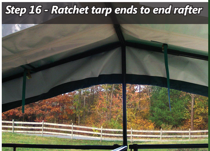
Step 16 - Ratchet tarp ends to end rafter
