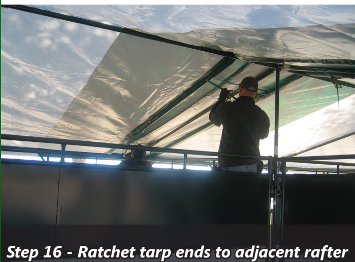
Step 16 - Ratchet tarp ends to end rafter
