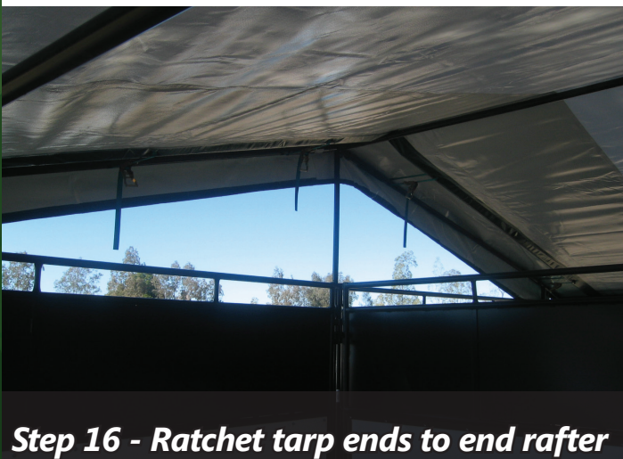
Step 16 - Ratchet tarp ends to end rafter
