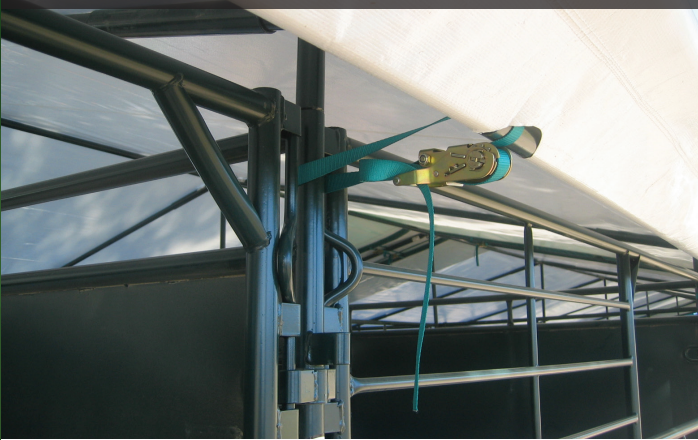
Step 15 - Ratchet eave securely to partition
