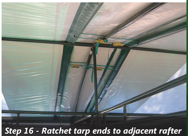
Step 16 - Ratchet tarp ends to adjacent rafter
